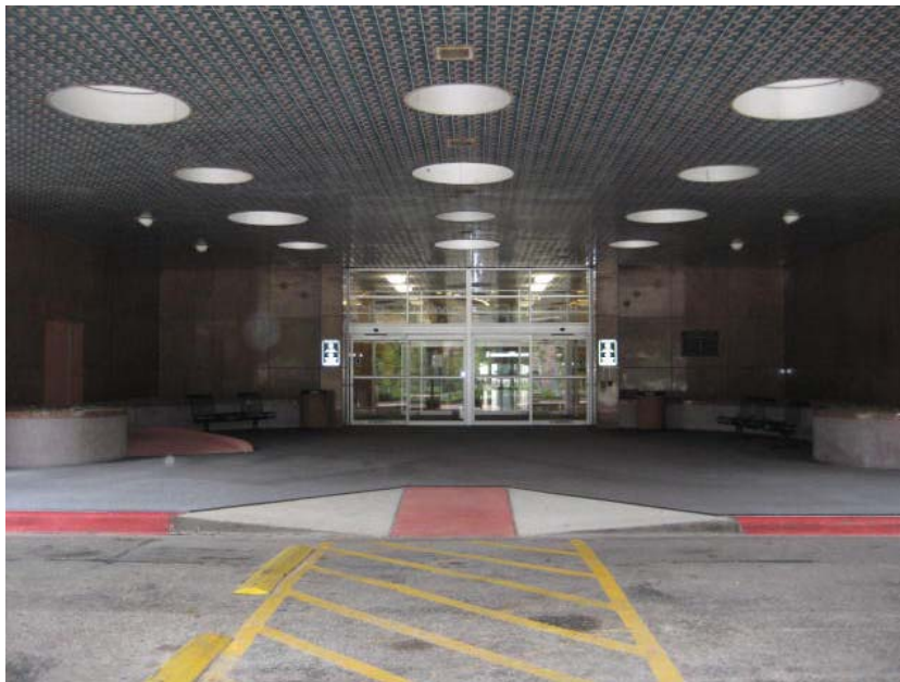
6. Underneath the building entry canopy where mural is to exit.
